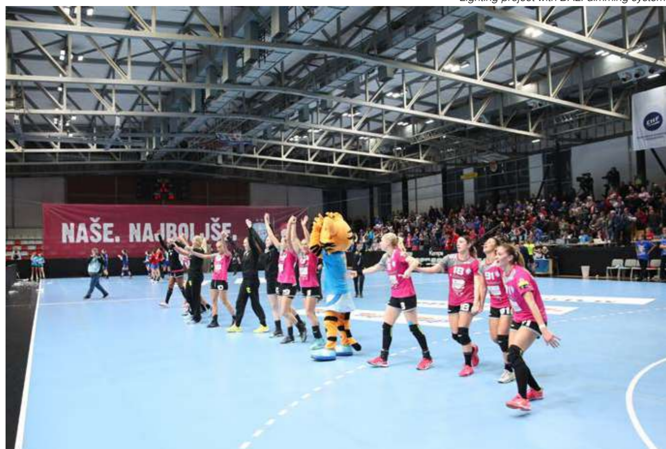
Lighting project with DALI dimming system.
